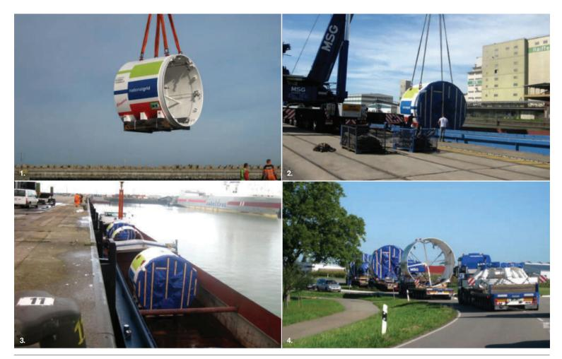
Specialist beam/vessel carrier trailers were used to transport the Shield with Main Drive, and the Machine Can with Erector. This method was chosen to enable the largest components to be safely carried beneath restricted bridge heights.
