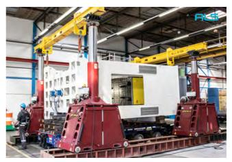
Specialist lifting equipment was used to position and install the unit utilizing a tower lift and set system from a heavy-lift Dutch manufacturer.
